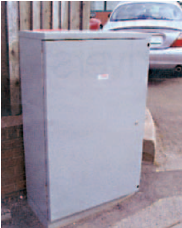
Above: As much processing as possible is done at the roadside. Right: a clear run of about 60metres is necessary to ensure that the driver will see the message.
