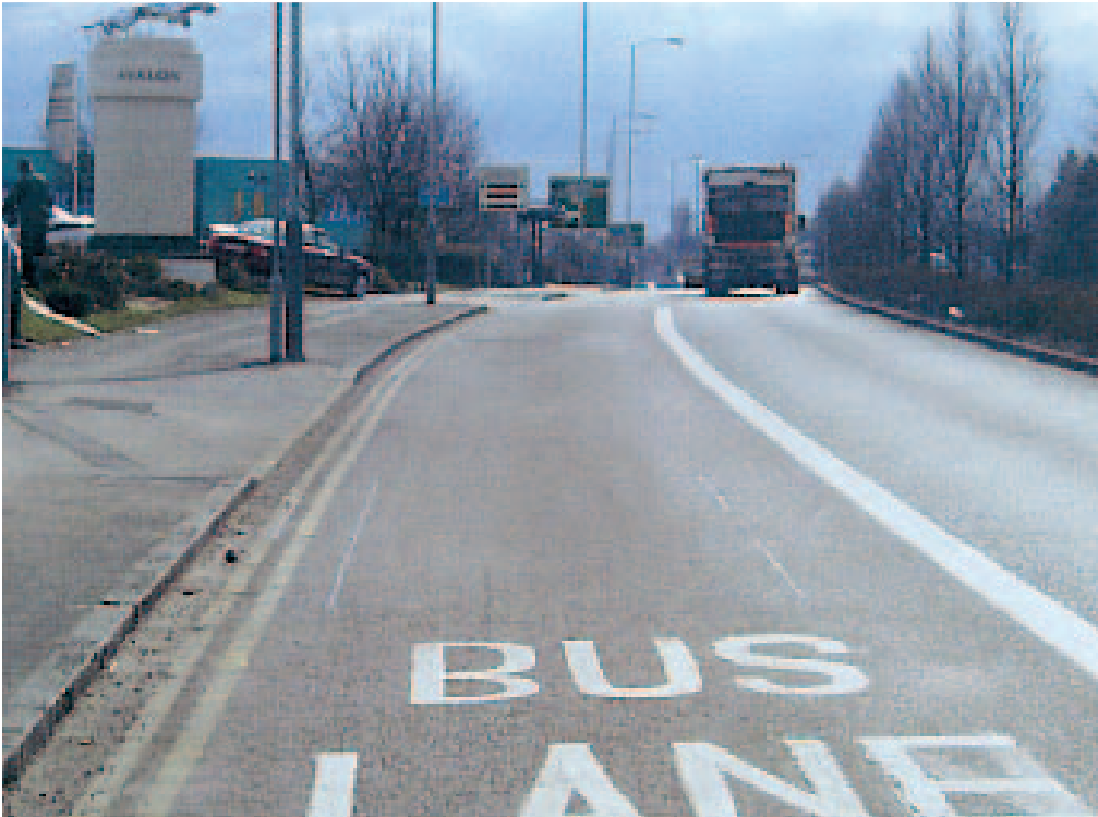
Above: As much processing as possible is done at the roadside. Right: a clear run of about 60metres is necessary to ensure that the driver will see the message.
